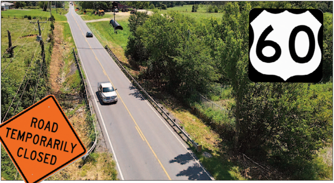
A culvert under US 60 in the foreground of this picture will be replaced with the black oval culvert sitting on the right side of the highway just past the guardrail.
